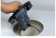
4. Place the FlexOn Gauge across the flange with the end flaps resting on the finished floor. The green area of the gauge, marked as TOILET HORN, should be pressing down and making contact with the inward seal. If the green area on the gauge barely touches or is above the sleeve opening, add more spacers as mentioned in Step 1.
