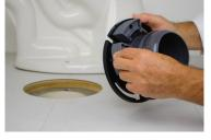
2. Wet the outer side of the sleeve. This will help it slide smoothly into the pipe at the time of installation.
